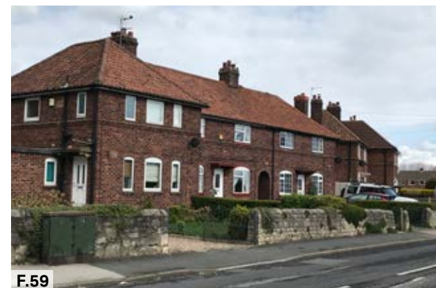
Figure 59: Red brick semi-detached dwellings along Ouston Ln
