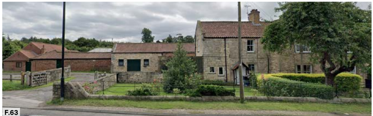
Figure 63: The Slip Inn Farm fronting York Rd and adjacent to the Turnpike Rd development
