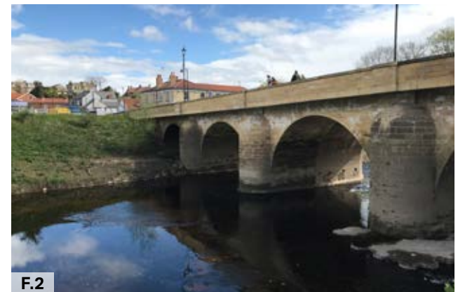
Figure 02: View of Tadcaster Bridge over the River Wharfe
