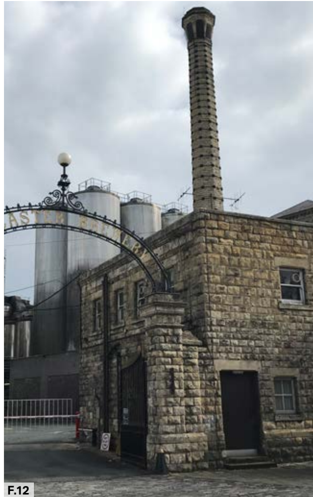
Figure 12: Chimney to John Smith's Brewery
